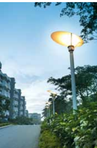
Product Design Pte Ltd installed 60 sets of Ligman 'Syndy Oval' 20641 indirect light using Philips 1 X 70W Master Colour CDMT Elite lamp source within the precinct of the Meadows@Pierce driveway. With its excellent colour quality, which remains stable through the product's lifetime, the installation ensures light output maintains display brightness at the lowest operating costs with low heat generation. Residents of Meadows@Pierce will have enhanced comfort as they walk or drive along the driveway.
