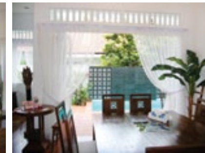
FAR LEFT: Instead of installing windows, French doors are incorporated in the interior, allowing natural winds to keep the home cool while giving it a very open and airy feel.
